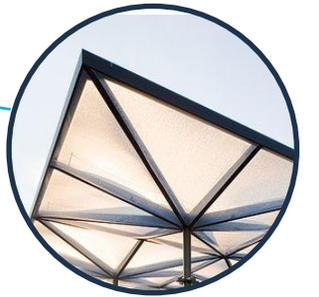
ETFE (Ethylene Tetrafluoroethylene) Clad Canopy
